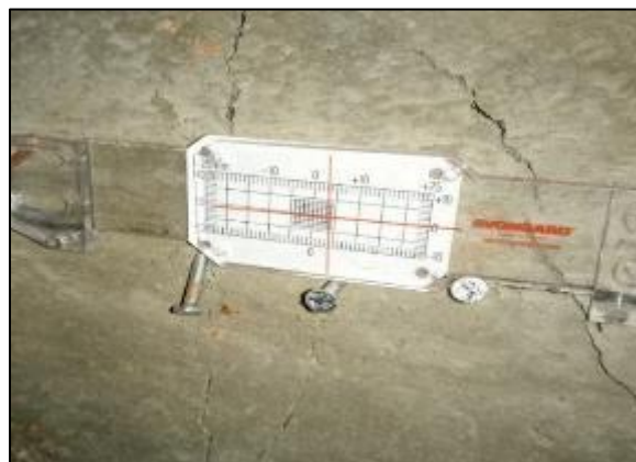
Figure 3 Crack pattern at failure for Beam 165×330
