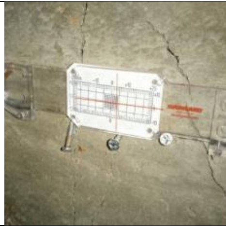
Figure 11 165 x 330 mm Deep Beam After loading to failure
