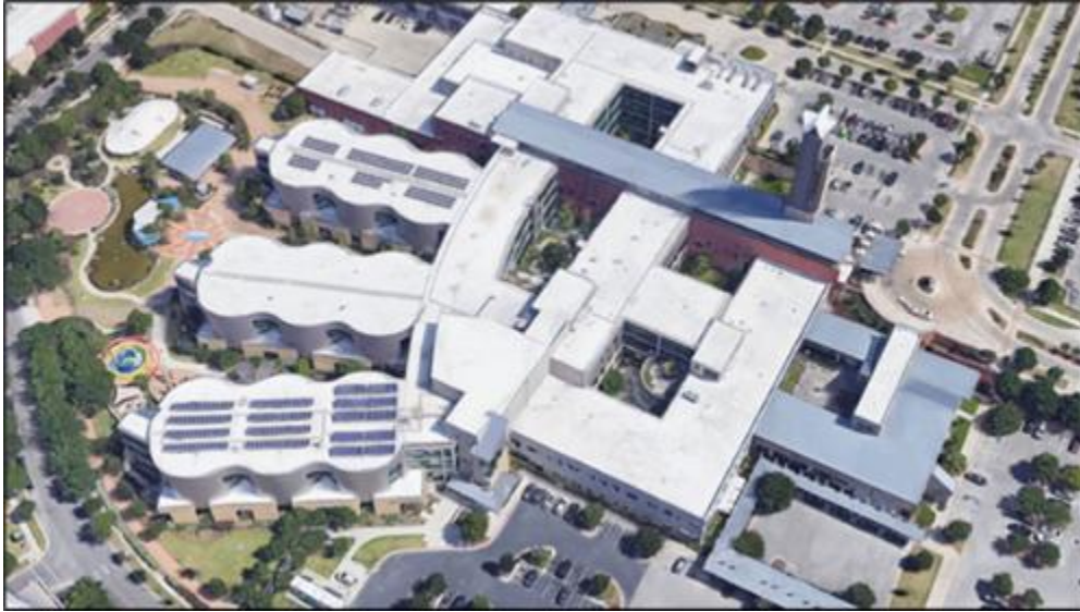
Figure 5 Dell Children's Medical Center, Austin, Texas, USA
