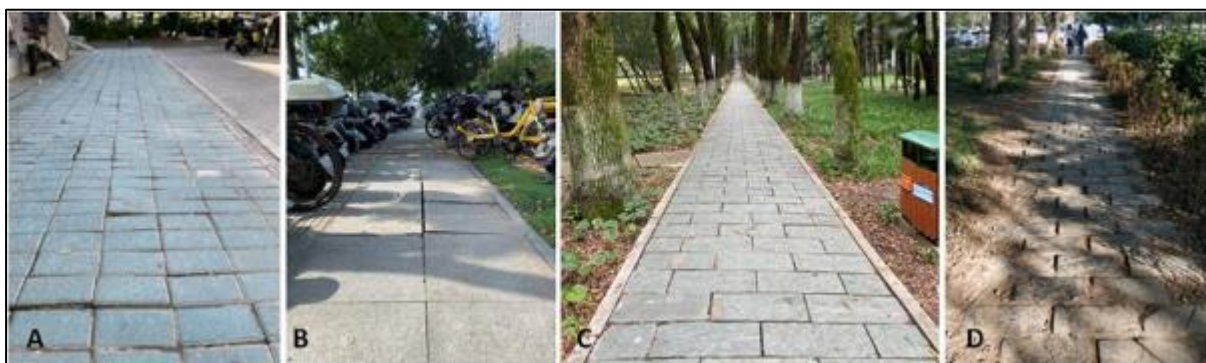
Figure 2 Walkways surface condition
