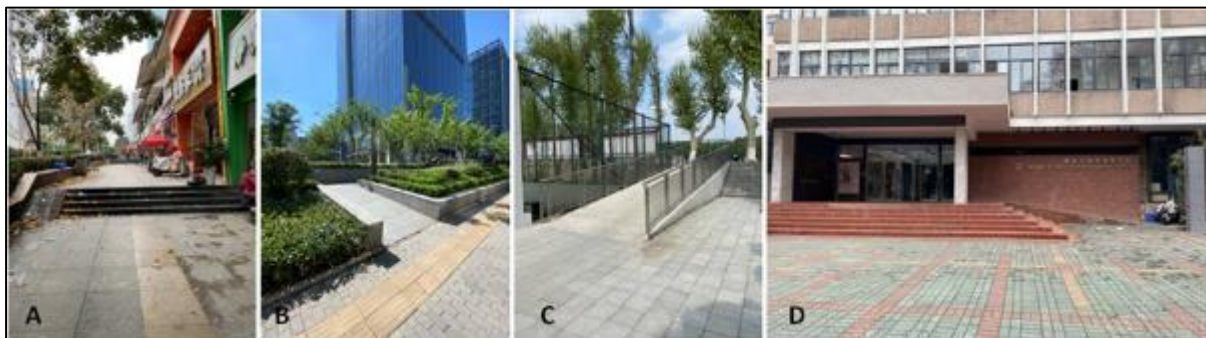
Figure 8 Buildings' entrances and public space ramps
