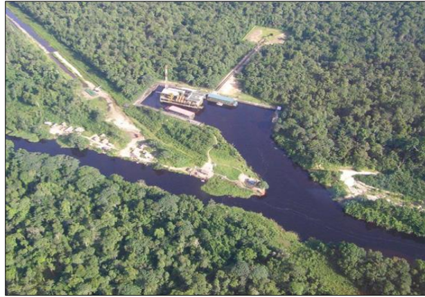
Figure 3 SSAGS, Ogbotobo site before construction
