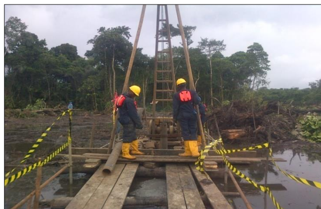
Figure 6 Bore Hole Drilling for Geotechnical Works at SSAGS Project location
