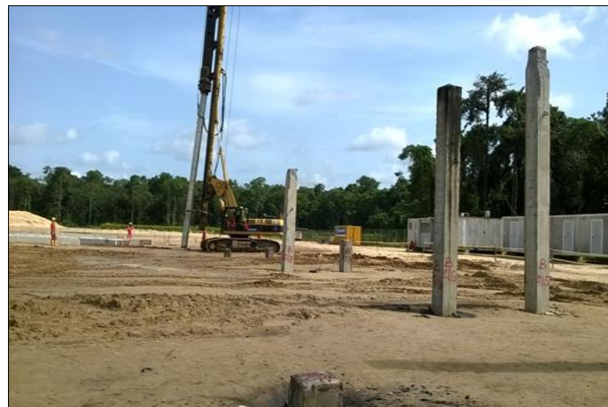
Figure 9 Piling operation at SSAGS Project Location
