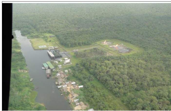
Figure 2 SSAGS, Opukushi site before construction
