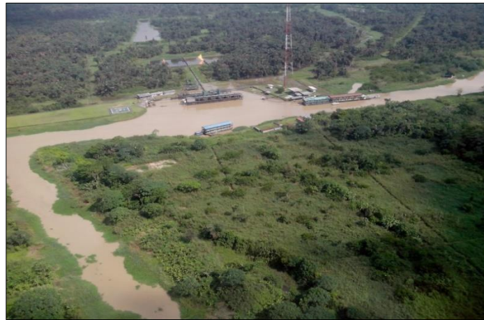
Figure 1 SSAGS, Benisede site before construction
