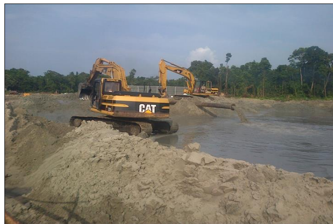
Figure 8 Dredging Operation of SSAGS Project Location
