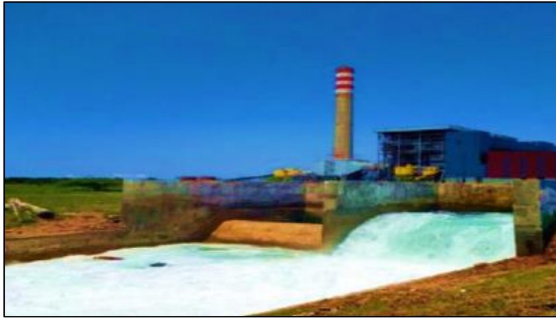
Figure 1 Outfall Condenser of Sebalang Power Plant
