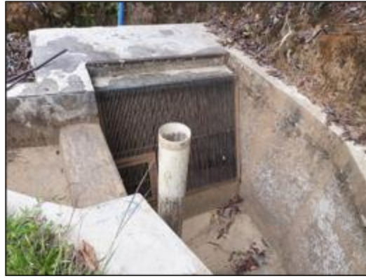
Figure 4 The condition of the forebay
