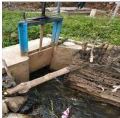
Figure 3 The condition of the intake
