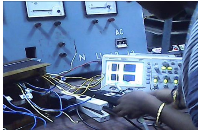
Figure 12 Hardware implementation test bed
