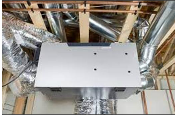
Figure 4 Solar Heater and Heat Exchangers
