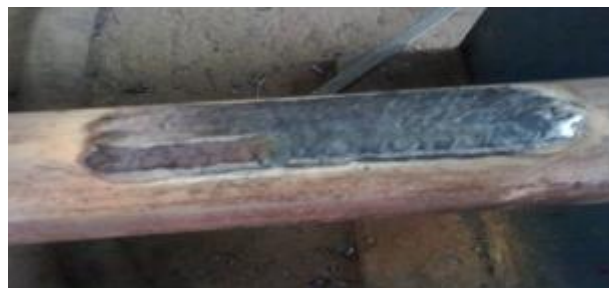
Figure 12 Tube surface after completion of post heating
