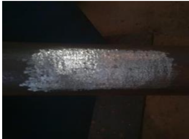
Figure 13 Tube Surface after grinding of excess deposition
