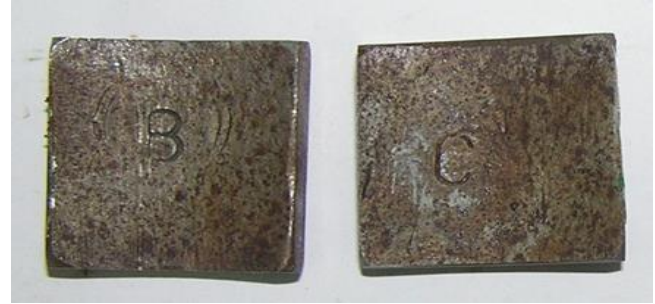
Figure 5 Corrosion on inner surface of sample B & C
