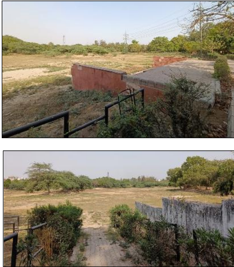
Figure 2 Existing site conditions
